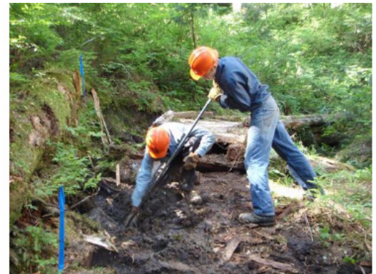
Courtesy photo Members of Northwest Youth Corps use a rock bar to move a stump during repair work on the Glacier Basin Trail on the northeast side of Mount Rainier National Park this summer.
